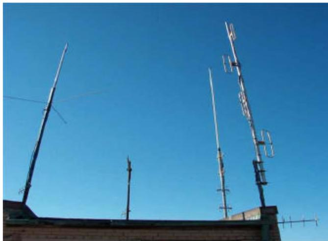
**Picture 1 — Four-Bay Folded Dipole on Right**
